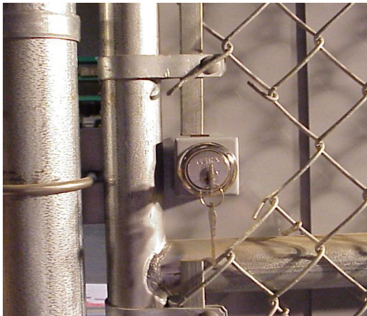
13. After latch bracket is adjusted properly, attach to post with tek-screws.
