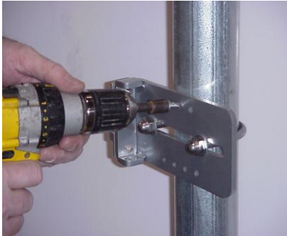
13. After latch bracket is adjusted properly, attach to post with tek-screws.
