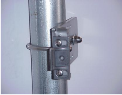
10. Screw strike latch to latch bracket.
